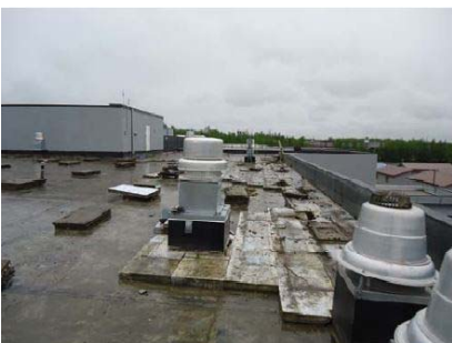
Roof B Wasilla, AK
