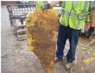
Roadway Insulation Minneapolis, MN
