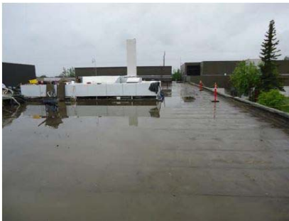
Roof A Wasilla, AK
