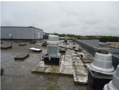
Roof B Wasilla, AK
