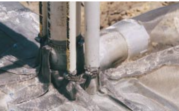
PHOTO 3: Termite mesh, a more recent development, is used to wrap the perimeter of the foundation or to prevent termites from gaining access through service penetrations. [Photo: Termi-Mesh Florida LLC]
