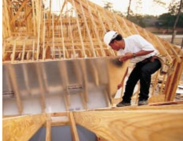
PHOTO 7: Protecting the structure by building with borate-treated wood products is a suppression option in certain situations. [Photo: Louisiana-Pacific® SmartGUARD™]
