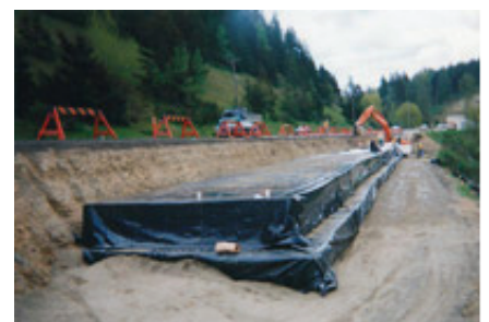
Figure 2 Installation of GeoSpec Lightweight fill Material
