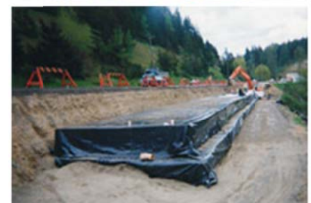
Figure 3 - Installation of GeoSpec Lightweight fill Material
